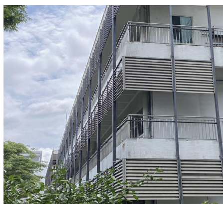
Figures 6 and 7: Different Blocks (S12 and S13) in the Science Faculty Look Remarkably Similar
